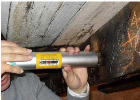
a. Pilodyn test in roof beam
