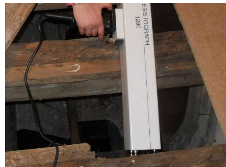
b. Resistograph in Pavement2 beam
