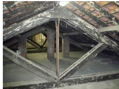
Figure 5 - Trusses of building 8
