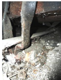
Figure 7 - Connection between timber truss and I beam through strips bolted to the web.
