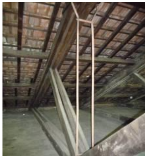
Figure 4 - Trusses of building 4
