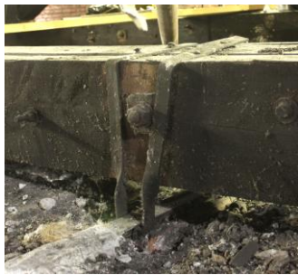
Figure 7 - Connection between timber truss and I beam through strips bolted to the web.
