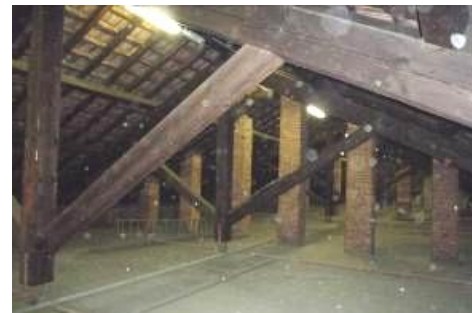
Figure 6 - Trusses of building 7
