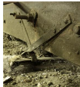
Figure 8 - Connection between timber truss and I beam through strips wrapped around the flange, with no bolting.
