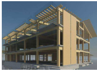
Figure 2a – The NMIT arts building with shear walls at both ends, and along the middle
