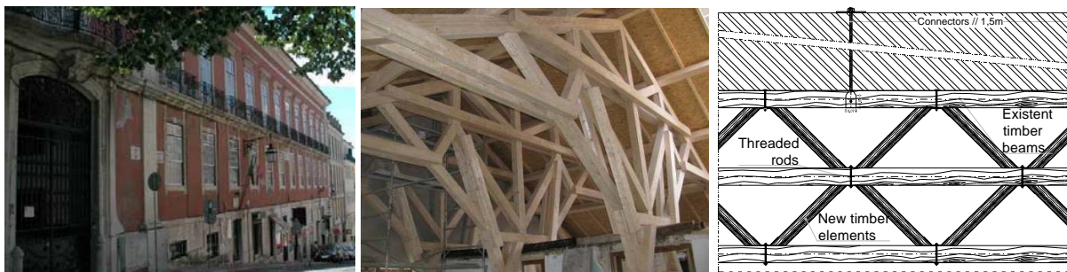
Figure 1 – Exterior photo of Valadares Palace and details of the structural intervention.
