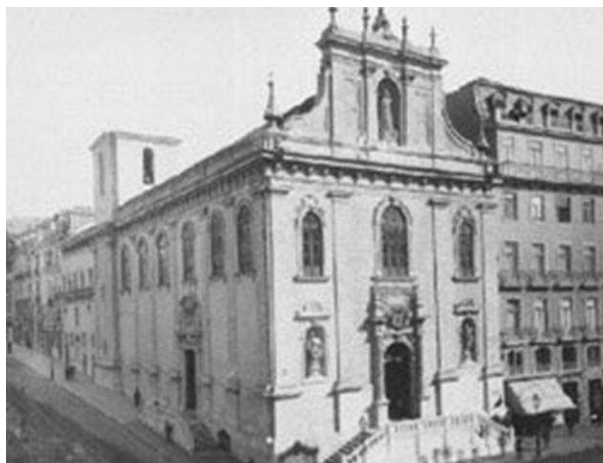
Figure 1 – Nossa Senhora do Loreto Church – South and West facade
