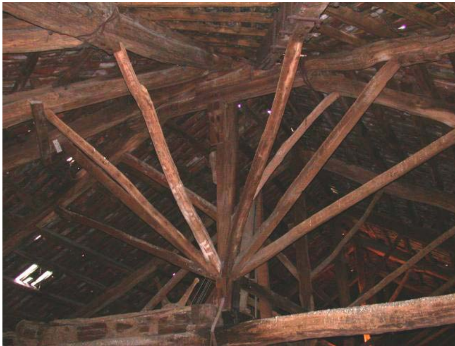
Figure 1 – Elements of the roof timber structure over the apse of the Cathedral of Vercelli Grading according to resistance
