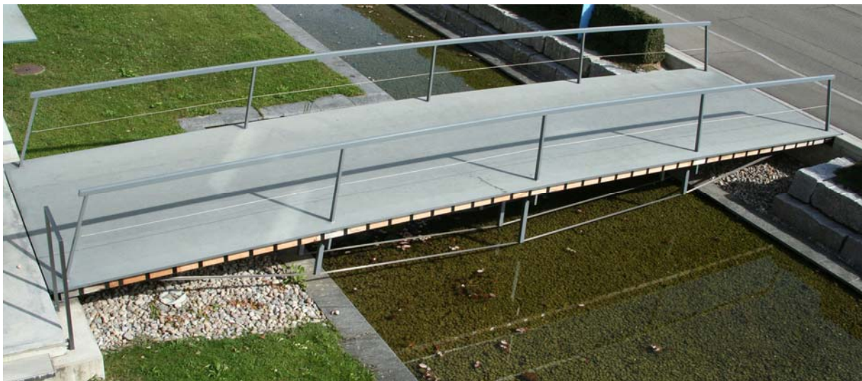
Figure 1 – Situation of the ready assembled bowstring arch bridge that spans over a pond at the Empa site in Dübendorf, Switzerland. The bridge is made exclusively of glulam, CFRP and GFRP elements and apart of the installed multi-sensor monitoring system does not contain any metal part. On top of the timber bridge plate a GFRP-decking is installed.
